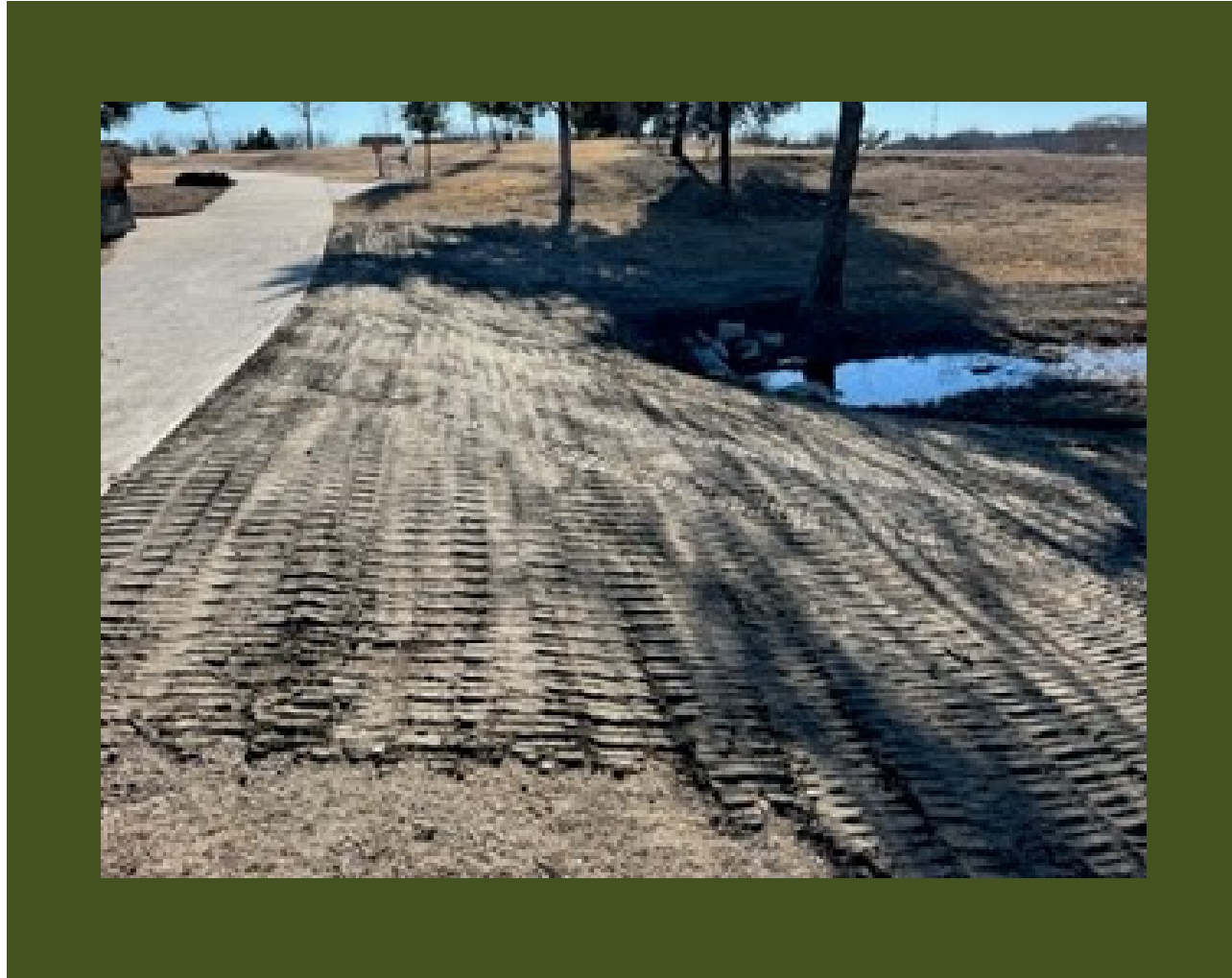
TCEQ HARRY MYERS DAM MAINTENANCE
