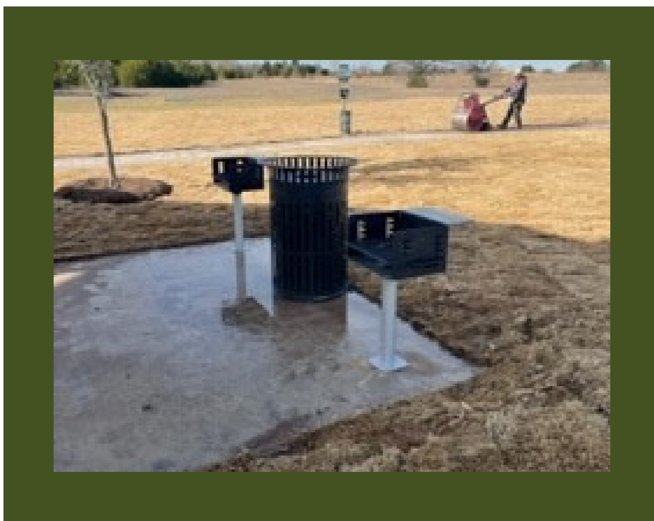
THE PARK AT TERRACINA BBQ GRILL INSTALLATION
