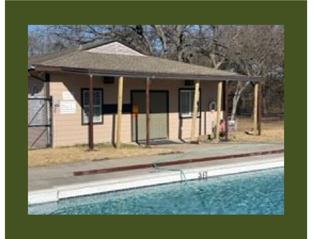
HARRY MYERS POOL BUILDING AWNING REBUILD
